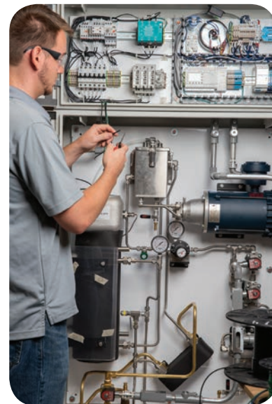
Assembling a system.
